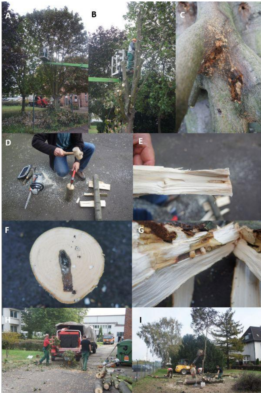
Figure 13: Time series of felling and processing infested trees. These trees must be felled in accordance with the phytosanitary measures required by Implementing Decision (EU) 2015/893: A) and B) Symptomatic trees (exit holes were discovered during monitoring) have to be felled; C) Additional symptoms (larval frass) become visible during the process; D) to G) Felled tree is dissected into smaller pieces, of which all must be inspected for living larvae, pupae and emerging adults; H) and I) All felled and inspected material must be chipped into pieces of not more than 2.5 cm in thickness and width (Source: Björn Hoppe)
